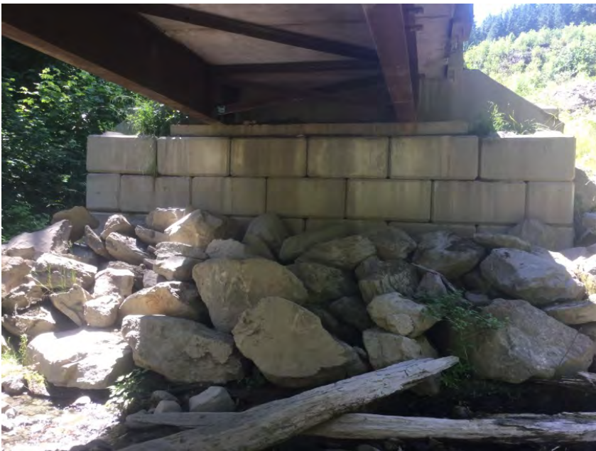
Right Bank Abutment when facing downstream
